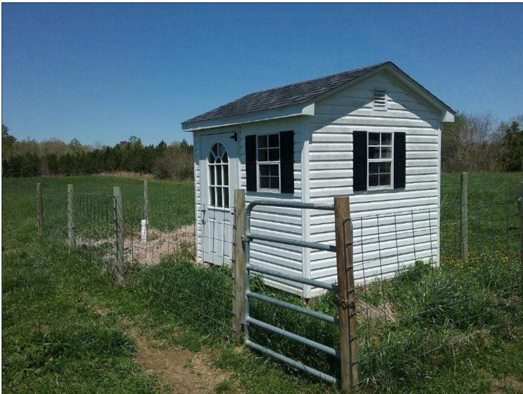
Figure 8-55: Standing structure in Area D2, facing north.
