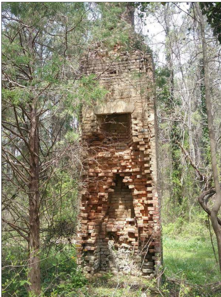
Figure 8-33: Inside of the standing chimney in Site 44LA0185.
